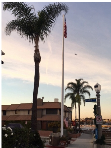
Sewer gas vent that holds a flag
